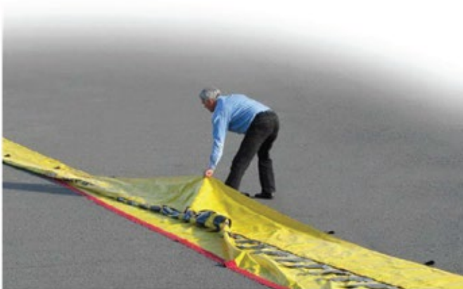
A - Completely unfold the Water-Gate.
