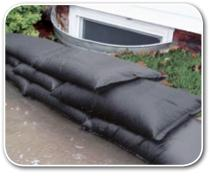
Brick & pyramid formation should always be stacked higher than water\* \*Jumbo Flood Bags can be stacked 4 high, if placed against a wall
